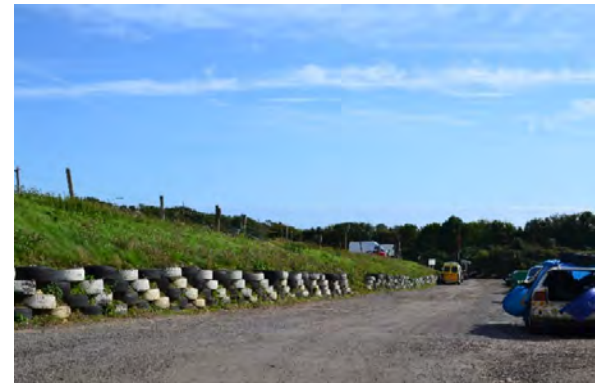
V8: Race track & bund wall
