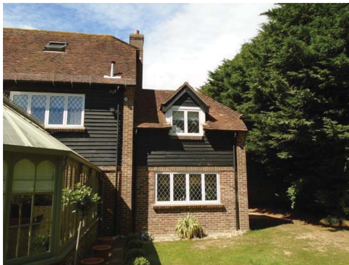
Building B1 - main house
