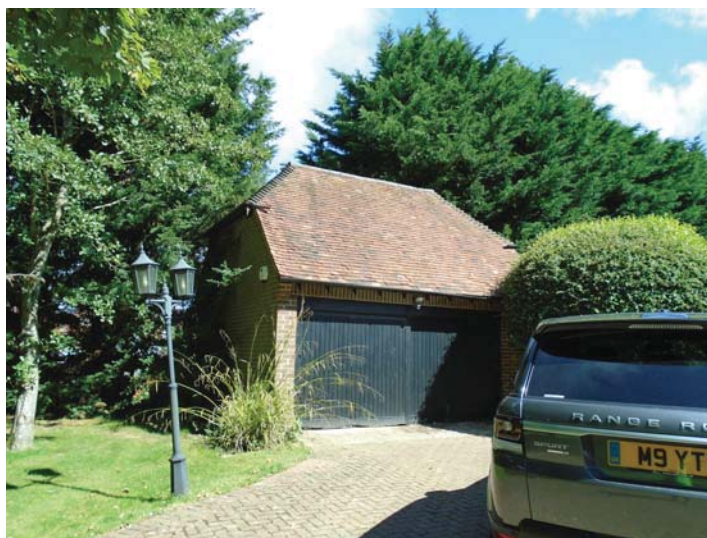
Garage building - B3
