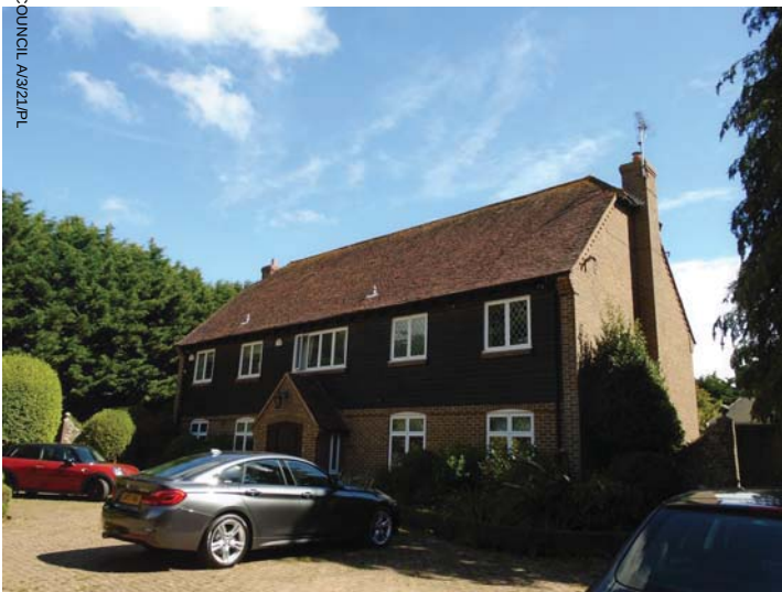
Building B1 - main house
