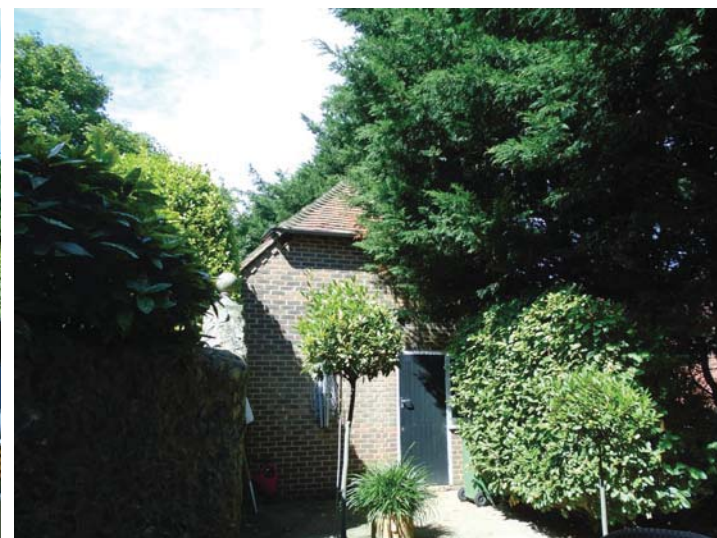
Garage building - B3
