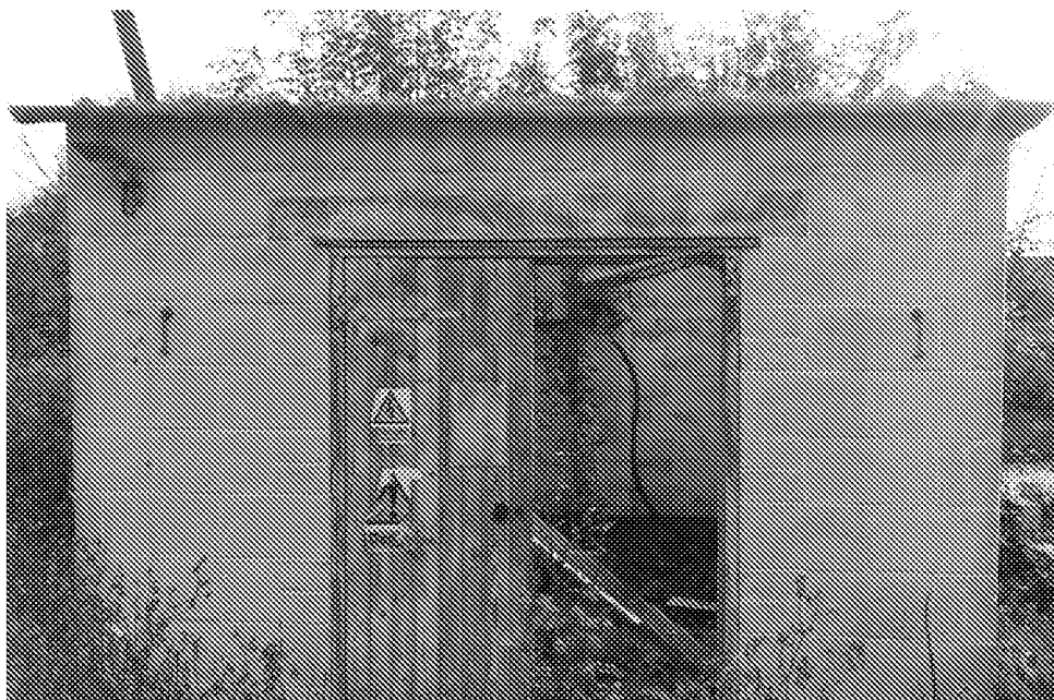
Photograph No. 15 - Building B1 which offered ' negligible ' bat roost potential.
