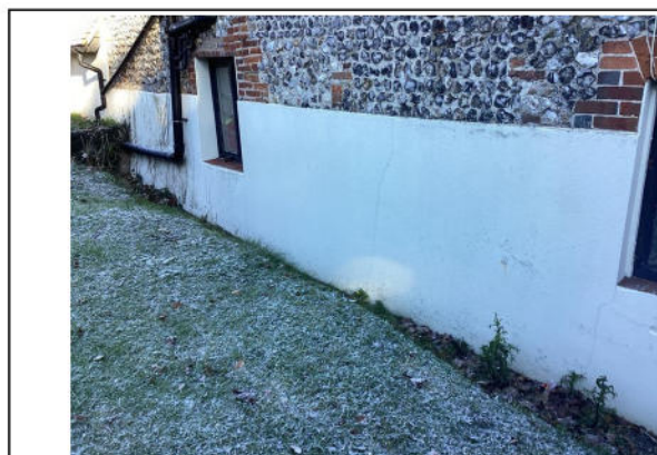
Sand and cement renders to the rear elevation
