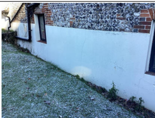
Sand and cement renders to the rear elevation
