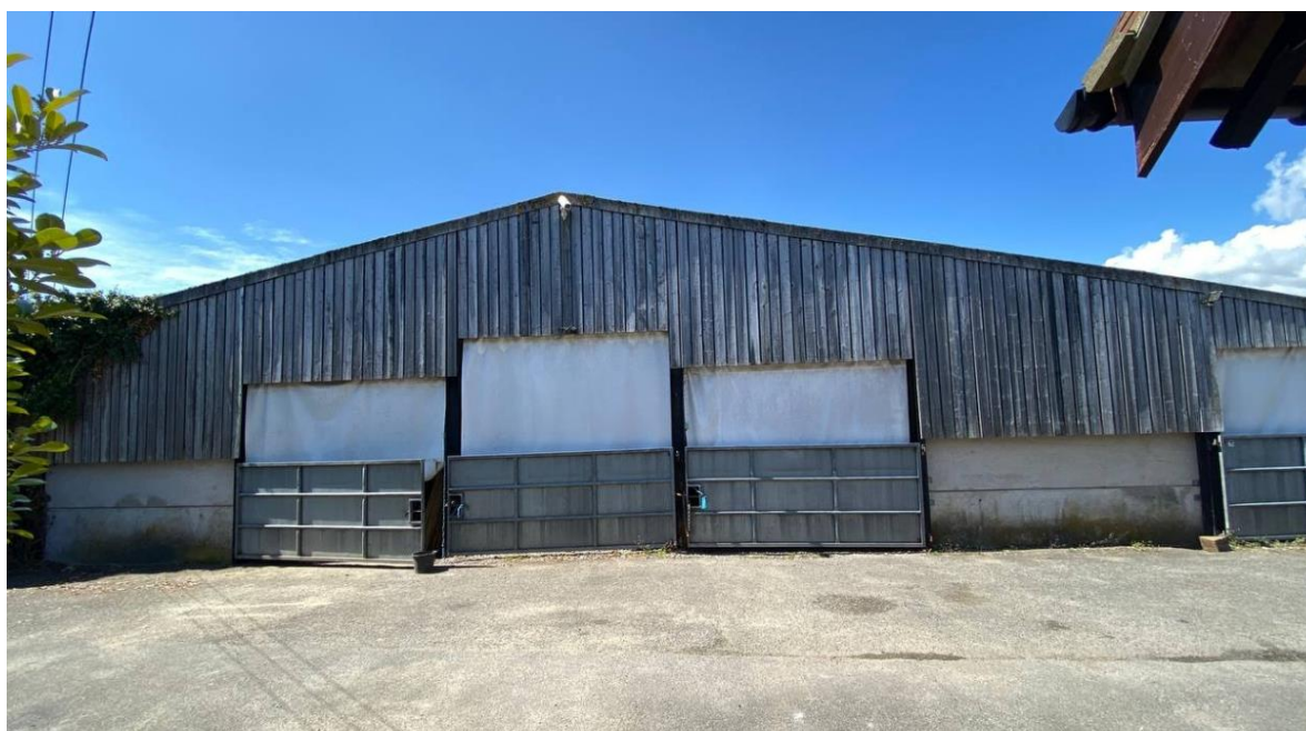
Figure 1- Barn as Existing (Eastern Elevation)
