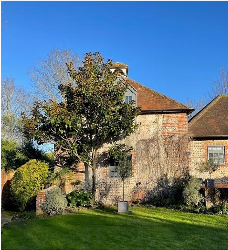
Figure 2- Dovecote at Ecclesden Manor (1353863)
