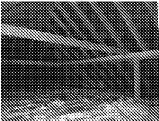
Plate 5. Loft of bungalow (B1)
