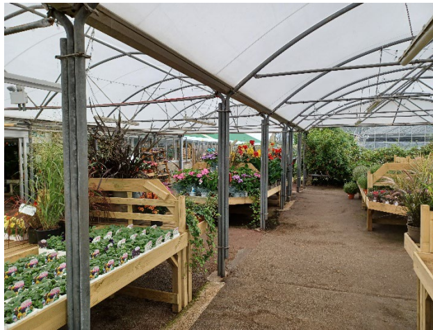
The existing canopy to be replaced.
