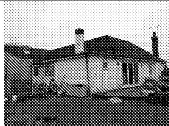
Photo 20: Northern and western elevations of Building B1.
