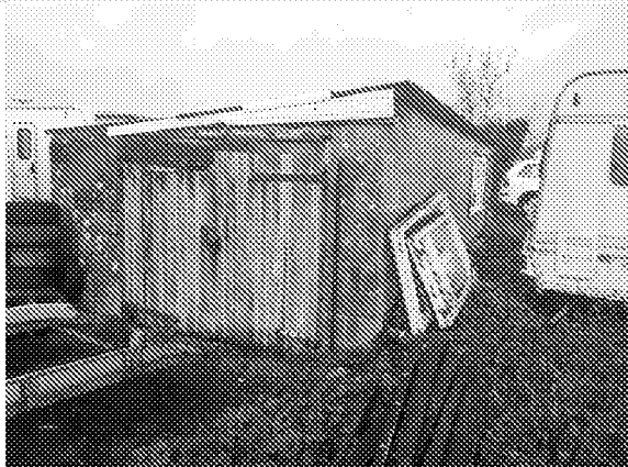
Photo 30: Building B7 looking north.
