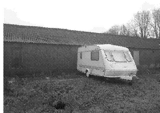
Photo 6: Eastern elevation of Building B10.
