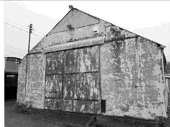
Photo 12: Western elevation of Building B3.
