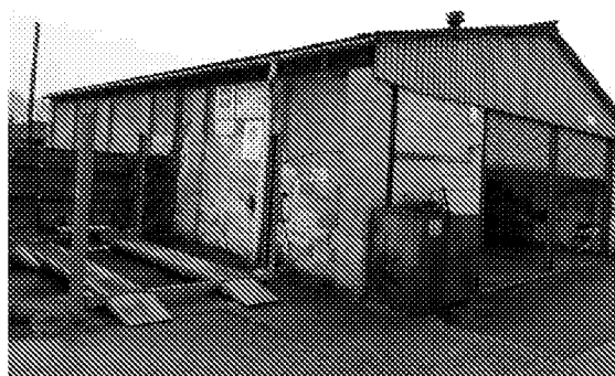
Photo 1: Southern and eastern elevations of Building B2.
