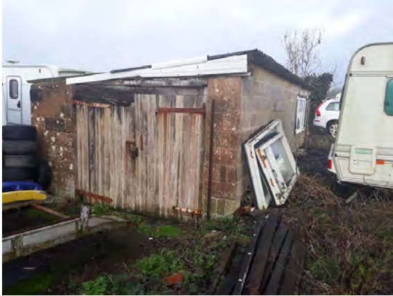
Photo 30: Building B7 looking north.
