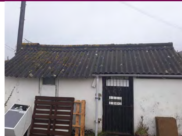
Photo 25: Southern elevation of Building B11.
