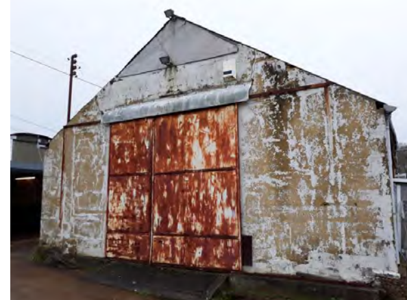
Photo 12: Western elevation of Building B3.
