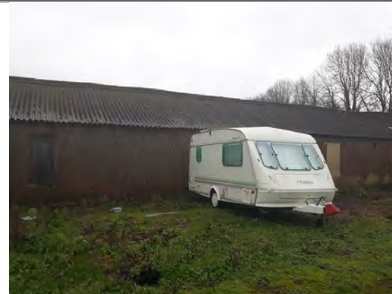
Photo 6: Eastern elevation of Building B10.
