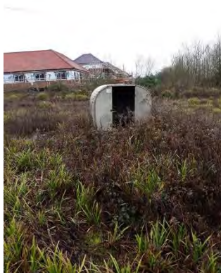
Photo 67: Building B14 looking east.
