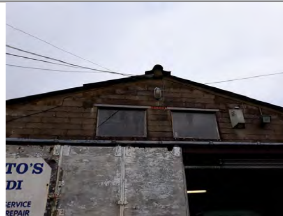
Photo 14: Southern elevation of Building B3 (previous bat roost in apex)
