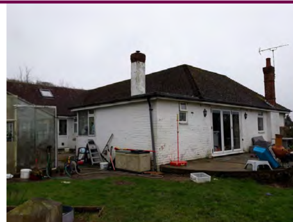
Photo 20: Northern and western elevations of Building B1.
