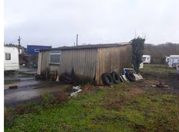
Photo 29: Building B12 looking south.
