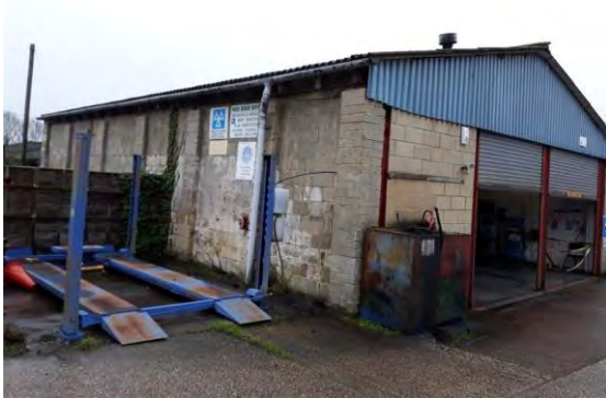
Photo 1: Southern and eastern elevations of Building B2.
