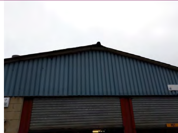
Photo 16: Eastern elevation of Building B2.
