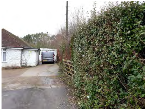
Photo 3: View looking east towards Building B1.
