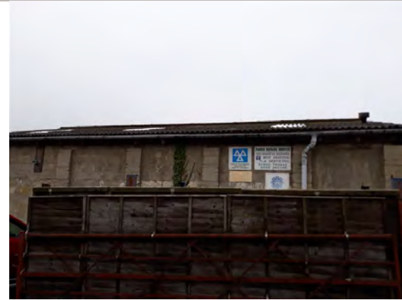
Photo 87: South western aspect of Building B1.
