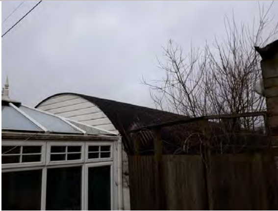
Photo 26: Northern elevation of Building B4.
