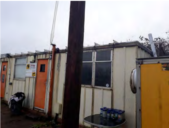
Photo 24: Western elevations of Building B12.
