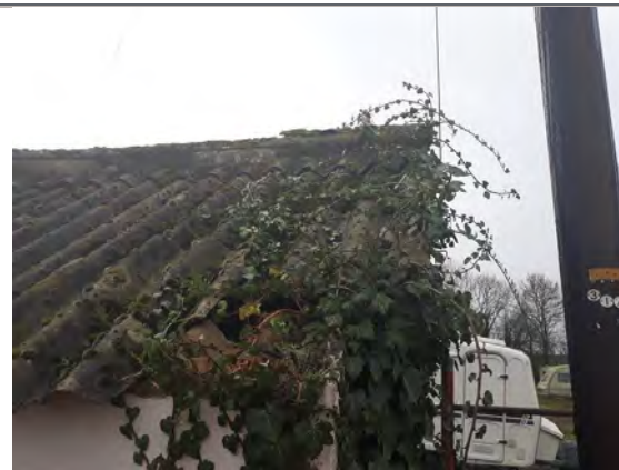
Photo 18: Southern elevation of Building B5.
