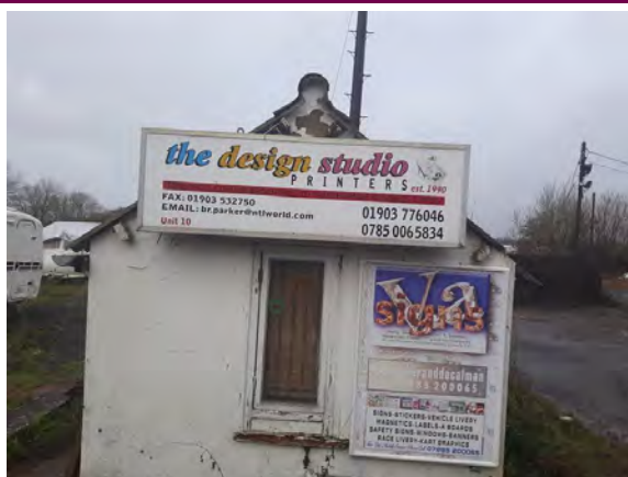
Photo 19: Eastern elevation of Building B5.
