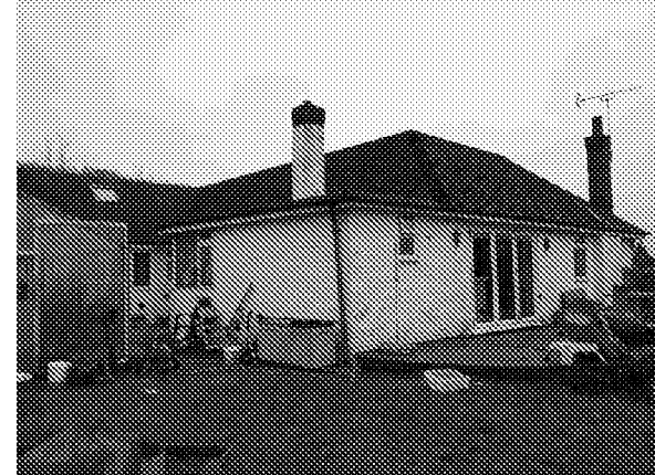
Photo 20: Northern and western elevations of Building B1.
