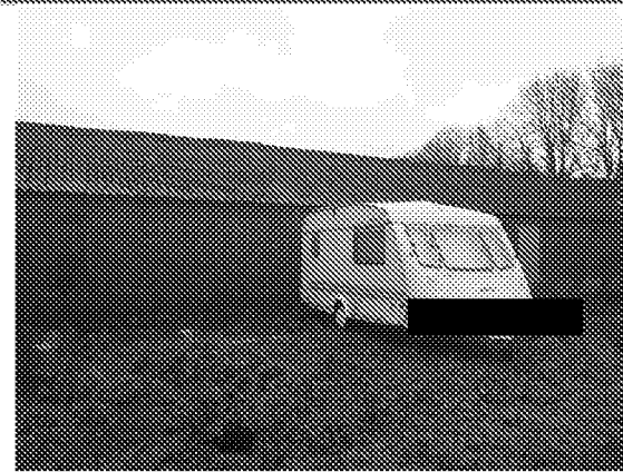
Photo 6: Eastern elevation of Building B10.
