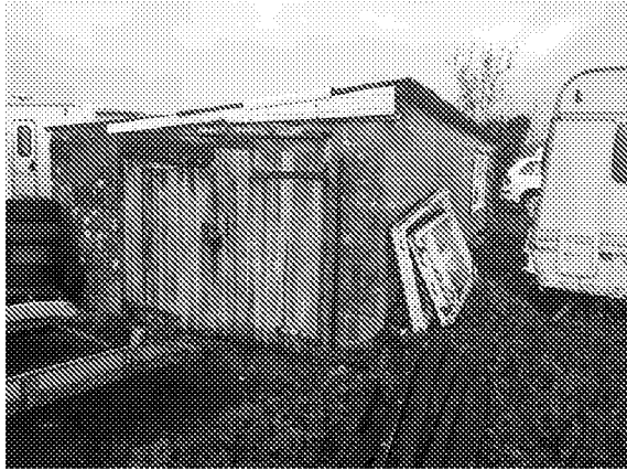
Photo 30: Building B7 looking north.
