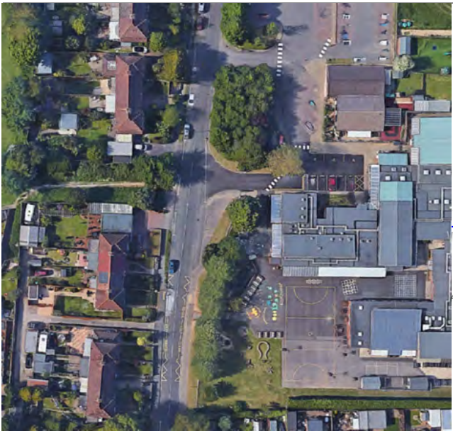
NORTH SOUTH AERIAL VIEW
