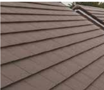
Red / brown roof tiles
