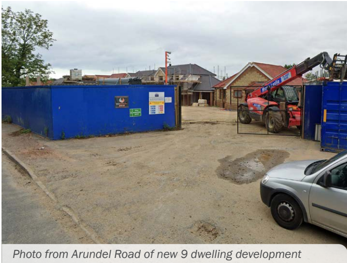
Photo from Arundel Road of new 9 dwelling development
