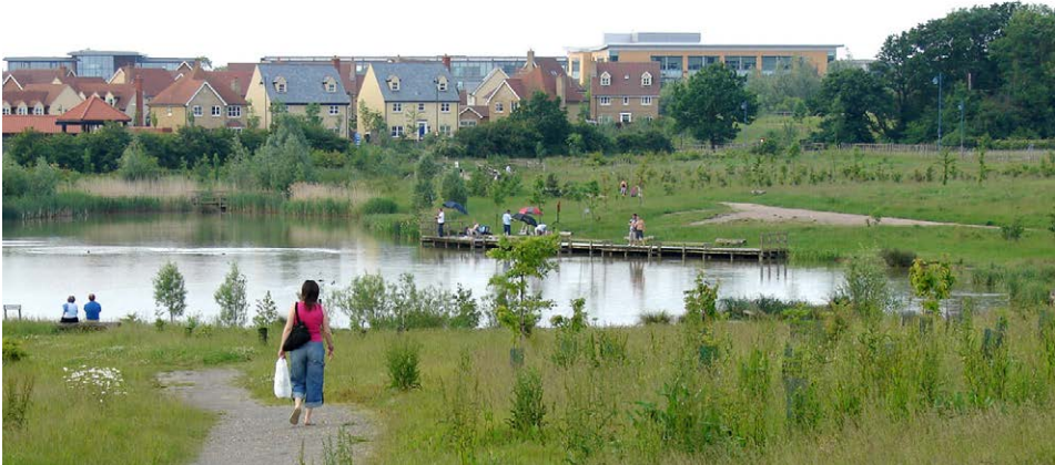
Planting designed for biodiversity and wildlife incorporated into SuDS infrastructure.
