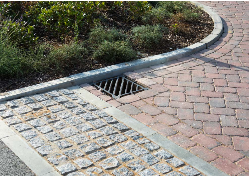
Permeable block paving and granite setts
