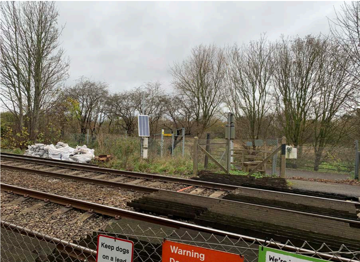
West Coast Railway line to south of site
