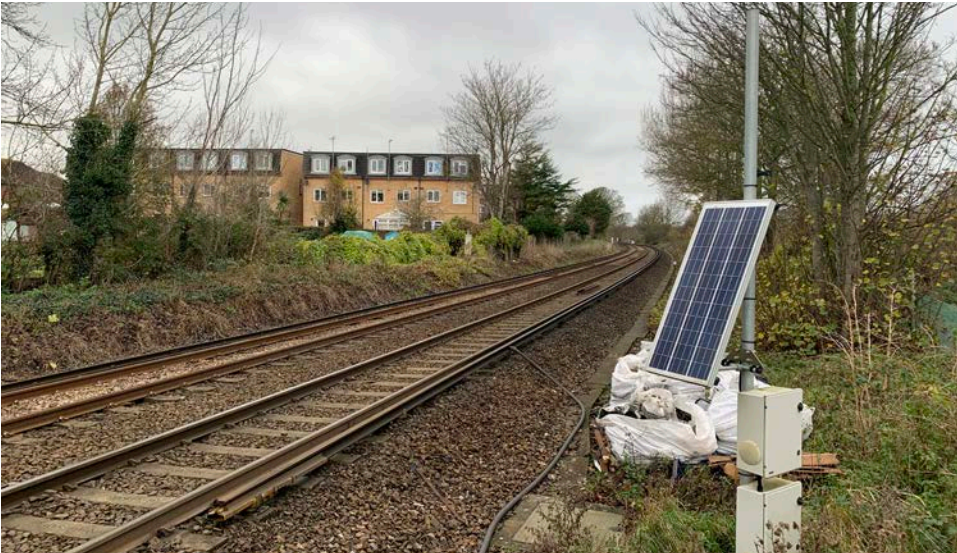
5. Railway to south at existing level crossing
