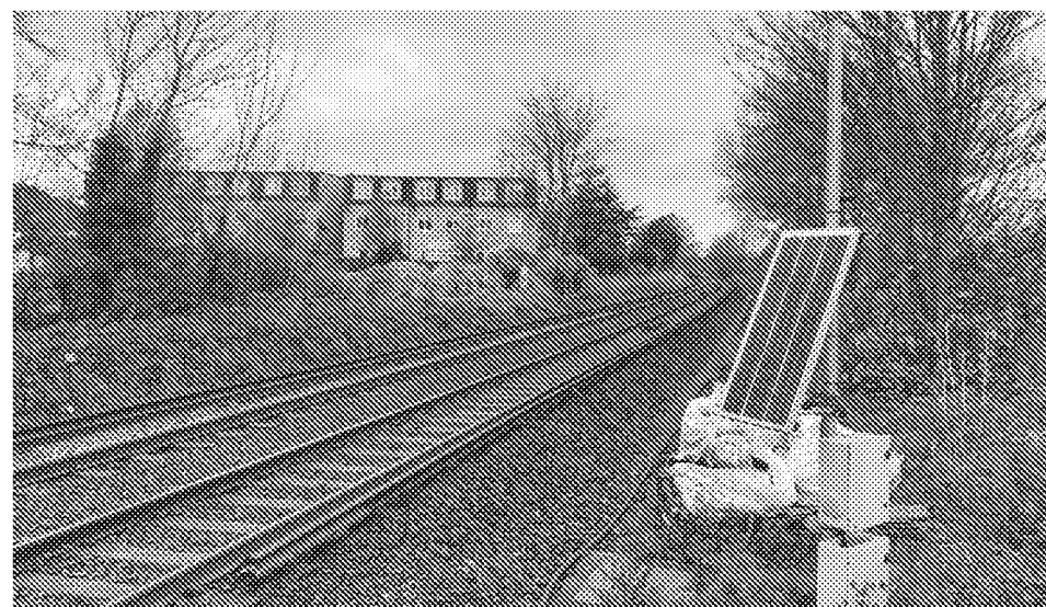
5. Railway to south at existing level crossing
