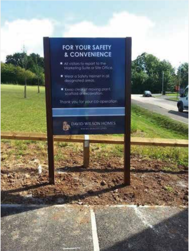
***PHOTO – TYPICAL INSTALLATION ***
