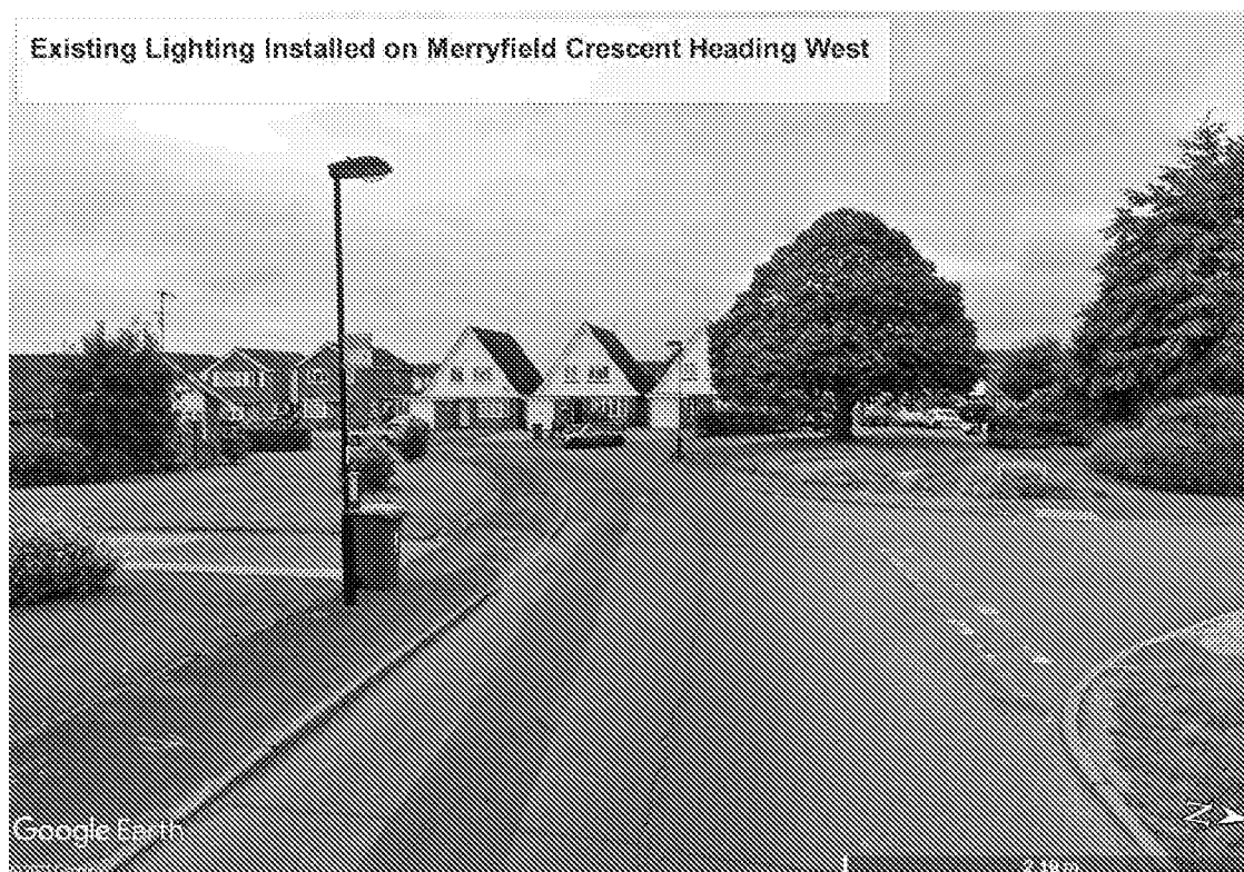
Figure 8 The existing lighting installed Merryfield Crescent heading west.
