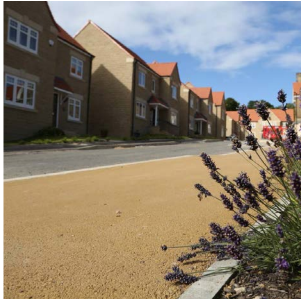
Buff coloured permeable surface to public footpath
