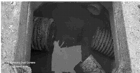
Figs 1, 2 - Pipes to be cut back to prevent being stepped on and chambers requiring sucking out of site debris
