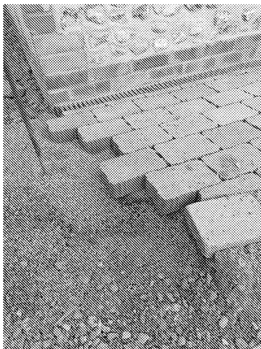
Figs 10 & 11 – Installation of permeable paving
