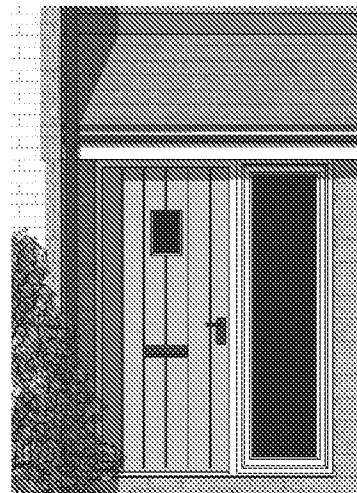
Lean-to pitched porch to front door
