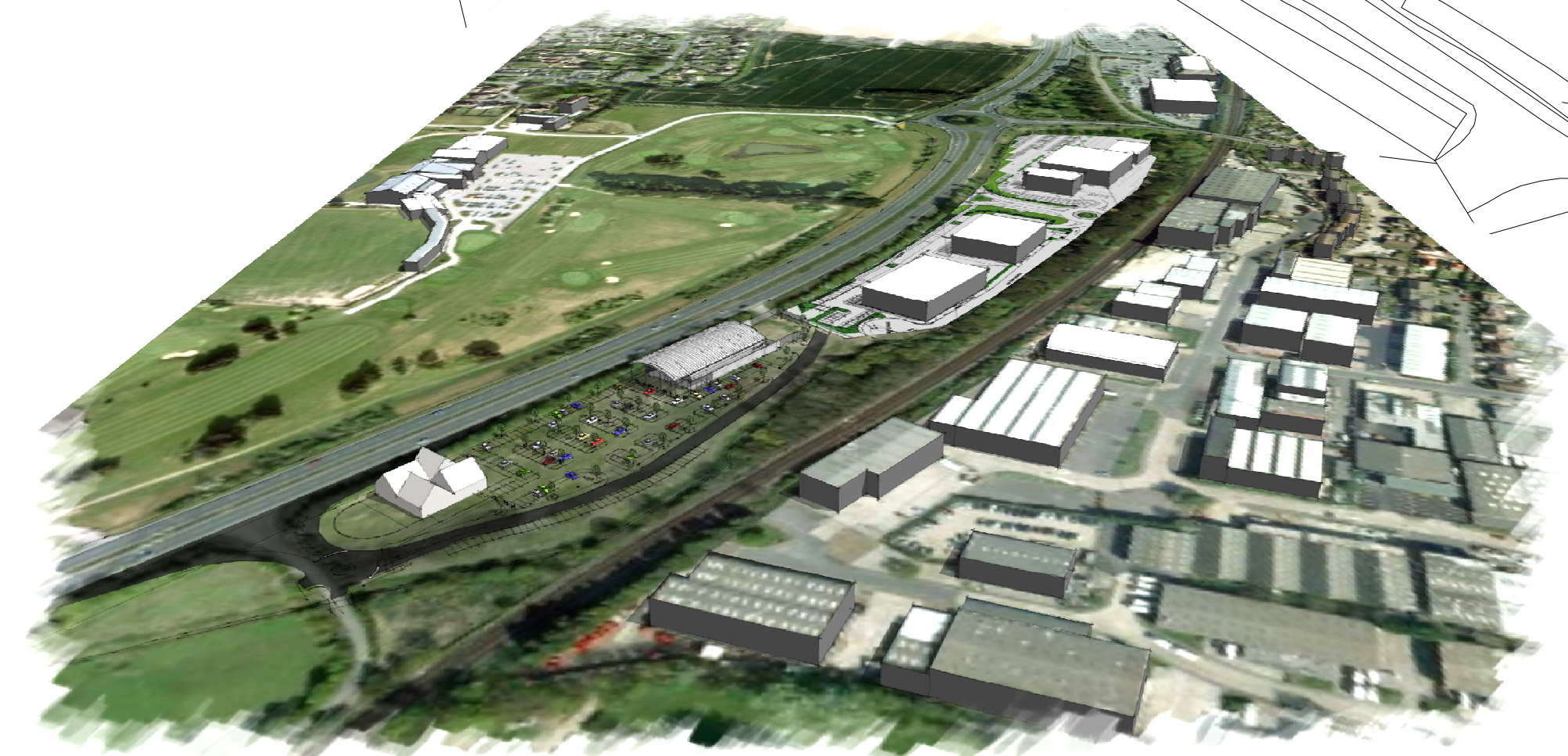
AERIAL VIEW FROM THE WEST
