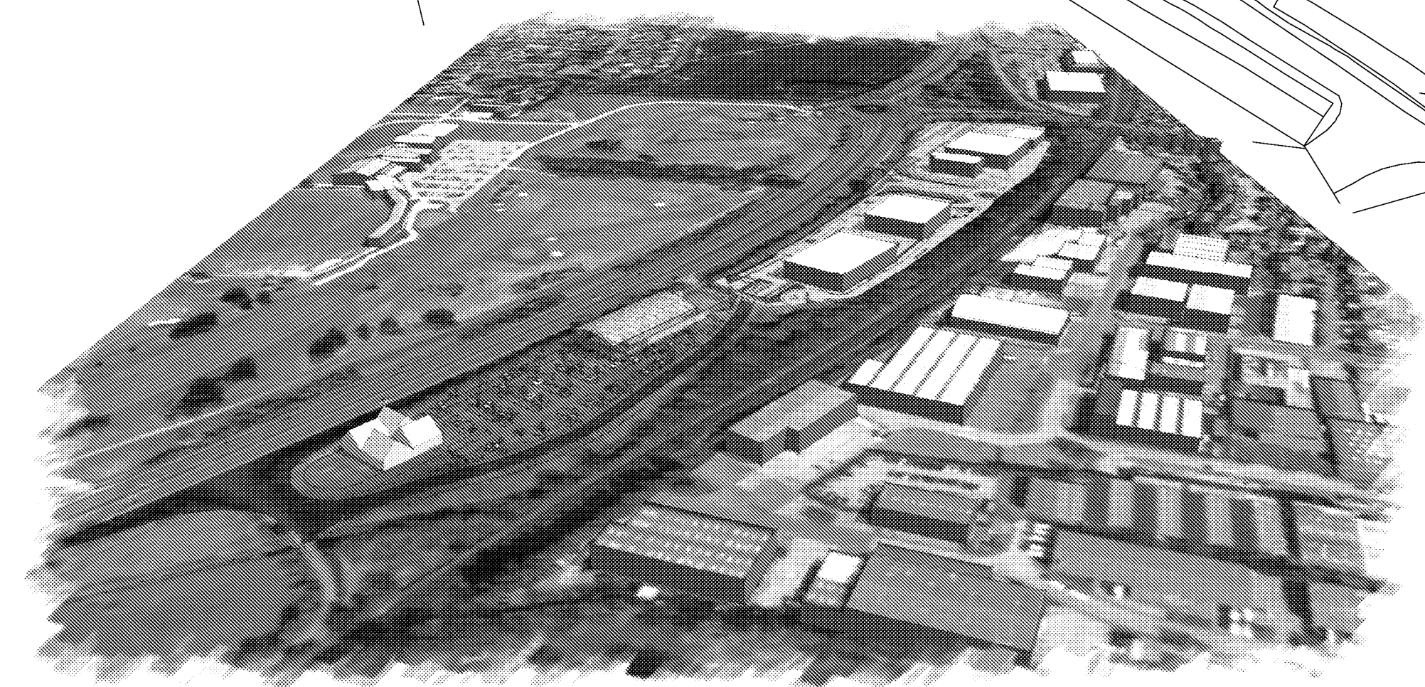
AERIAL VIEW FROM THE WEST
