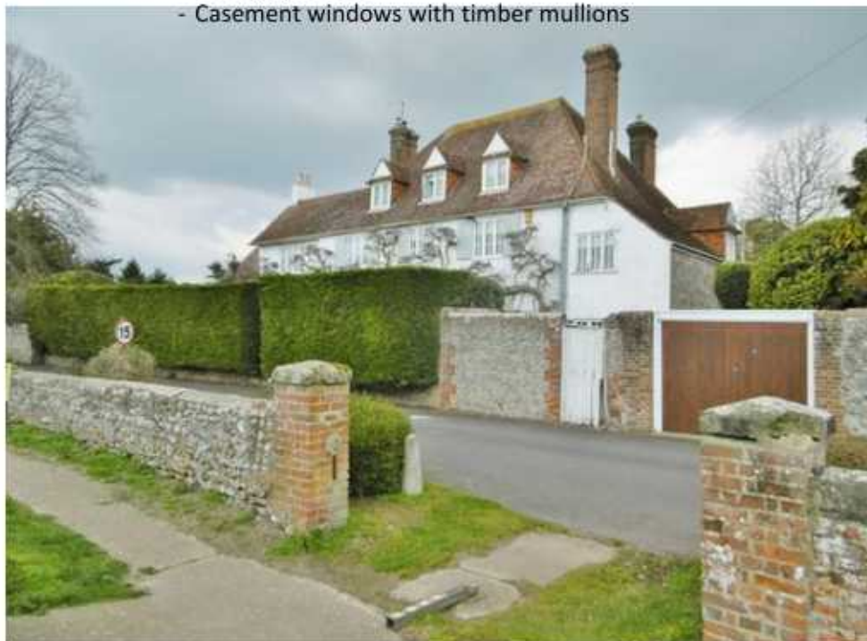
Front elevation including the extension at the end. Only the roof is minimally perceptible from Rectory Lane.
