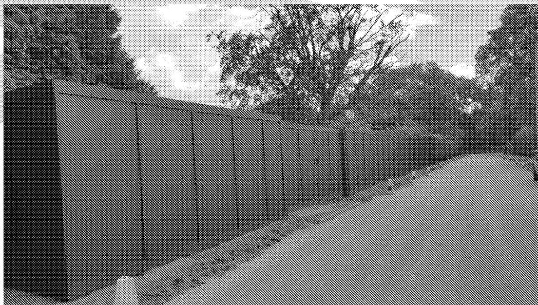
Timber hoarding with locked timber gate
