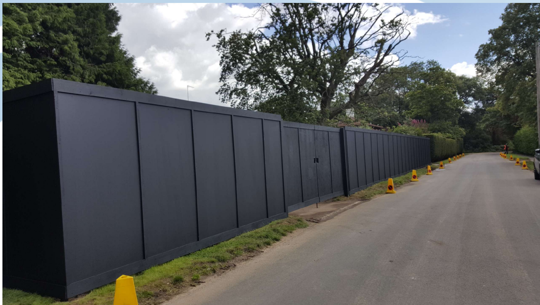
Timber hoarding with locked timber gate
