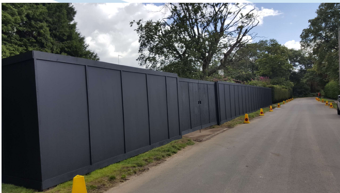
Timber hoarding with locked timber gate
