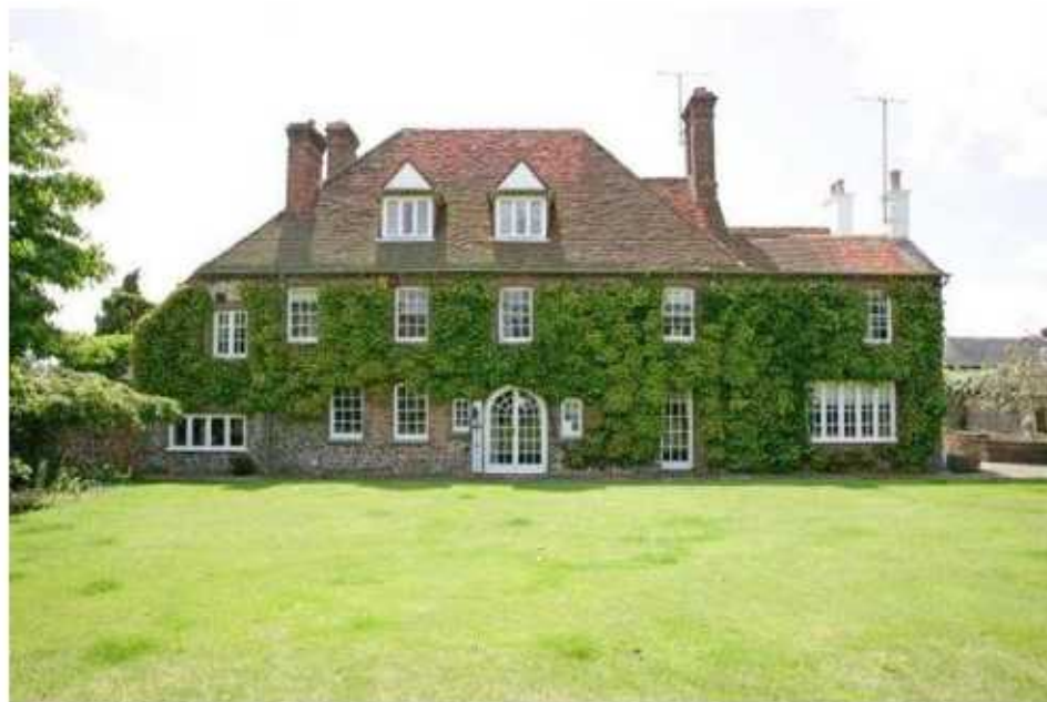
Existing rear elevation (from the rear garden)
