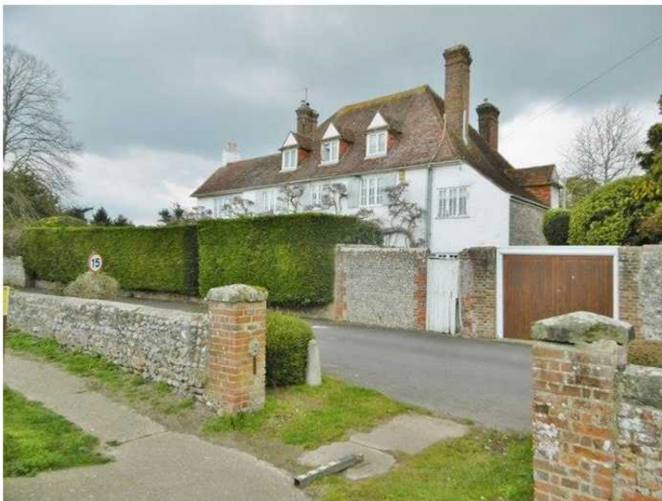
Existing front elevation (Rectory Lane)
