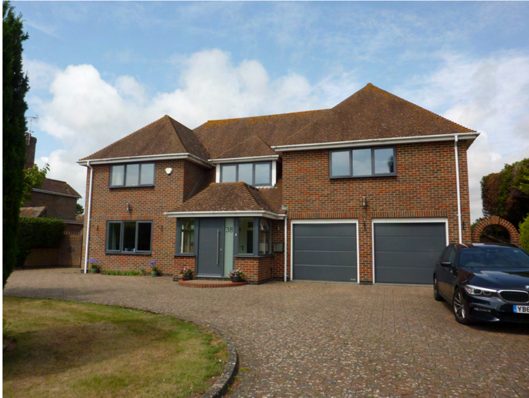
Photograph of front Elevation
