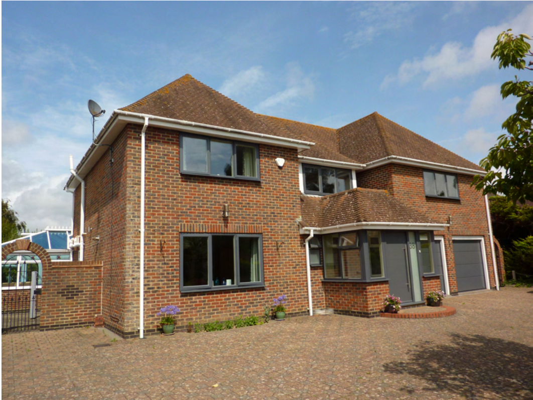
Photograph of front Elevation
