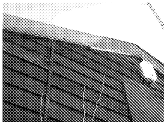
Photograph 8. Cobwebbed gaps between grooves of timber cladding and bargeboard (north elevation).
