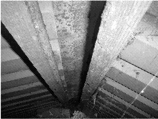
Photograph 13. Unlined roof with exposed ridge (Roof Void 1).
