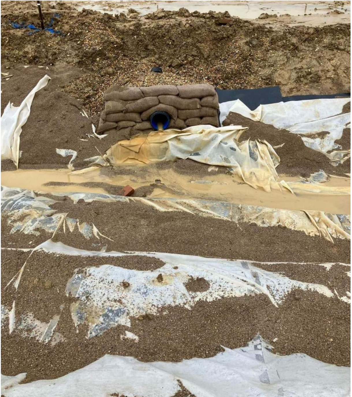
Photo of Concrete Bagwork Headwall During Construction
