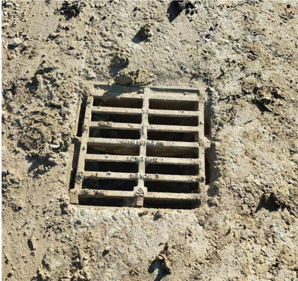
Road Gully Installed on Site
