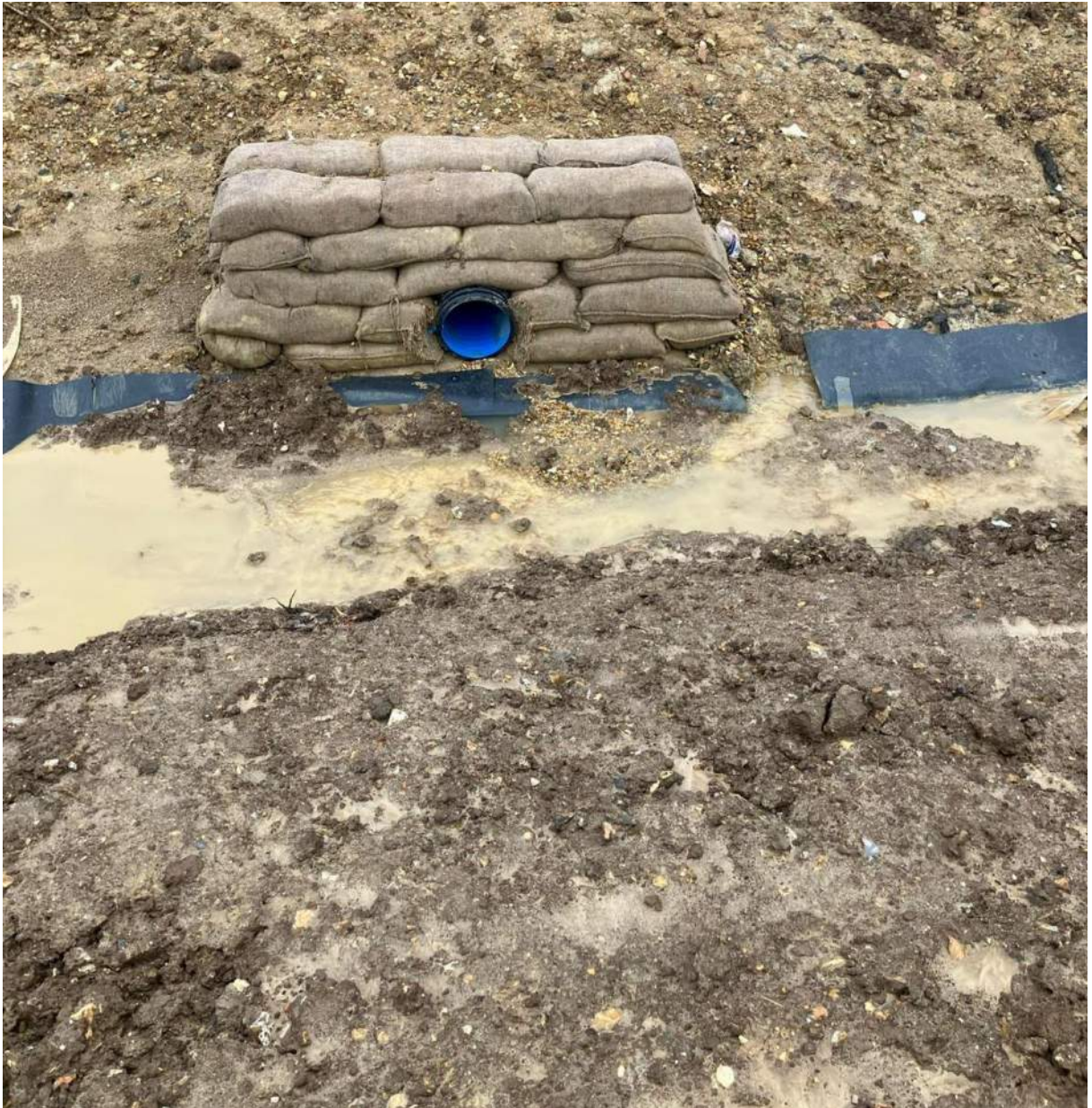
Photo of Concrete Bagwork Headwall During Construction
