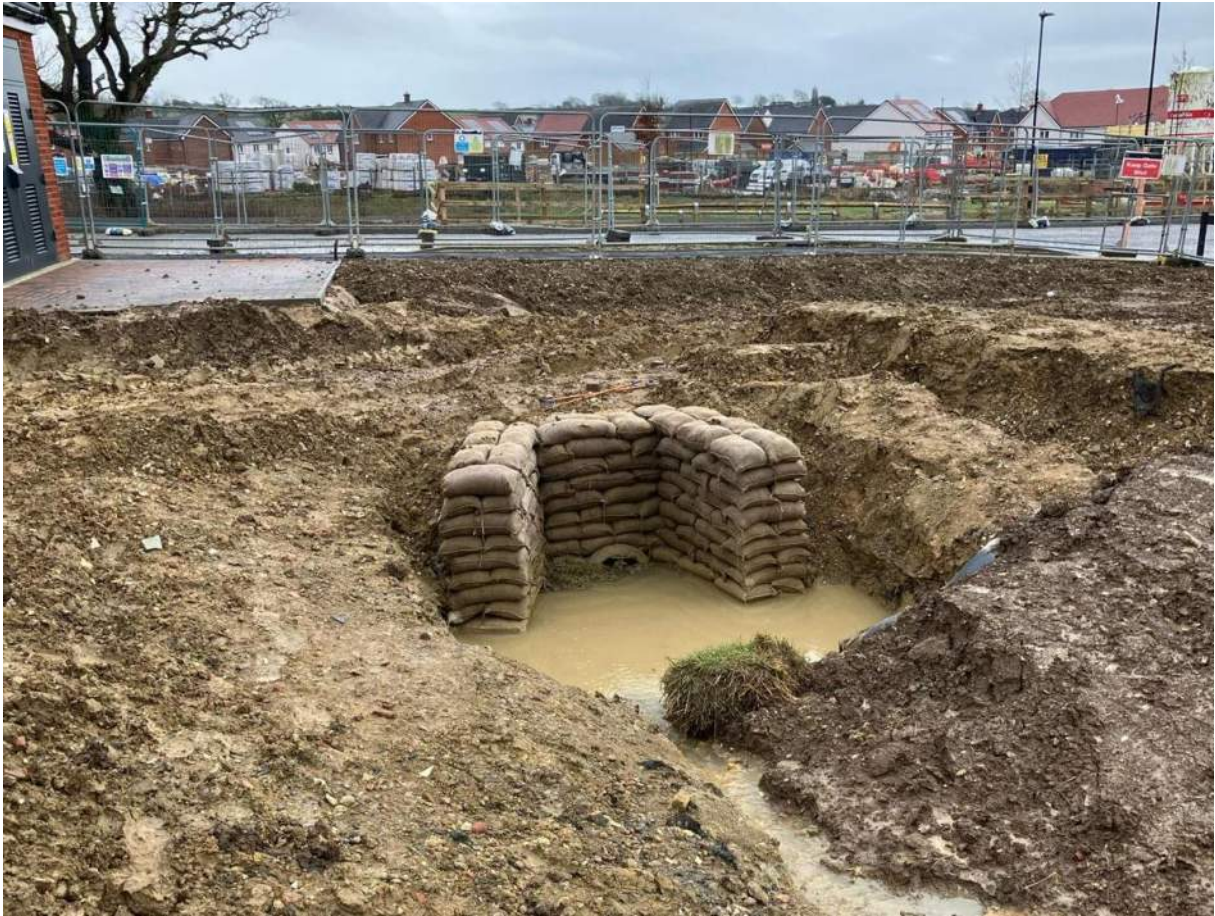
Photo of Concrete Bagwork Headwall During Construction
