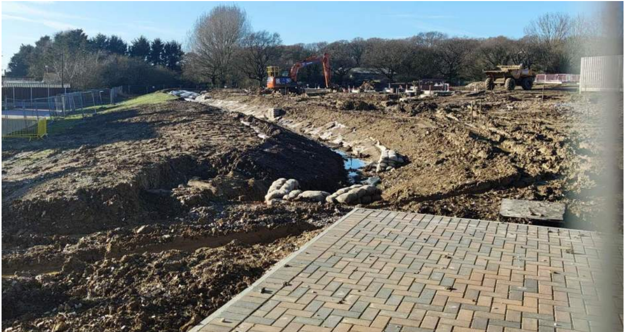
Swale During Construction
