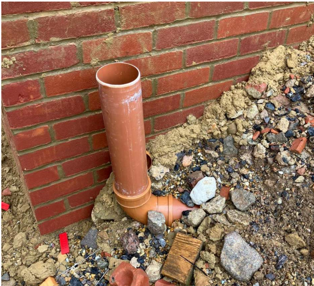
Photo of Rainwater Pipe During Construction
