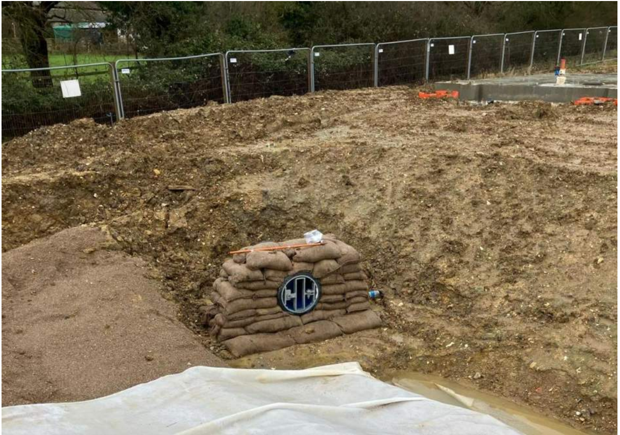
Photo of Concrete Bagwork Headwall During Construction
