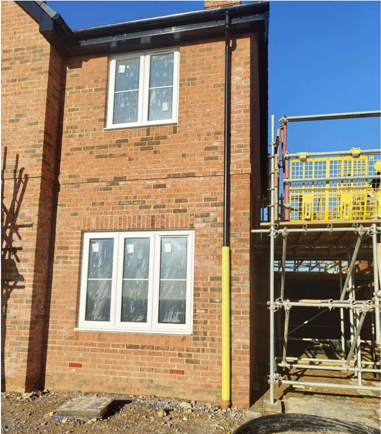
Rainwater Pipe Installed on Site
