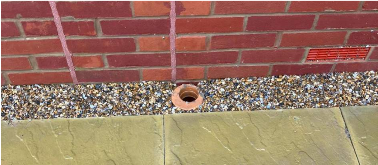
Photo of Rainwater Pipe During Construction
