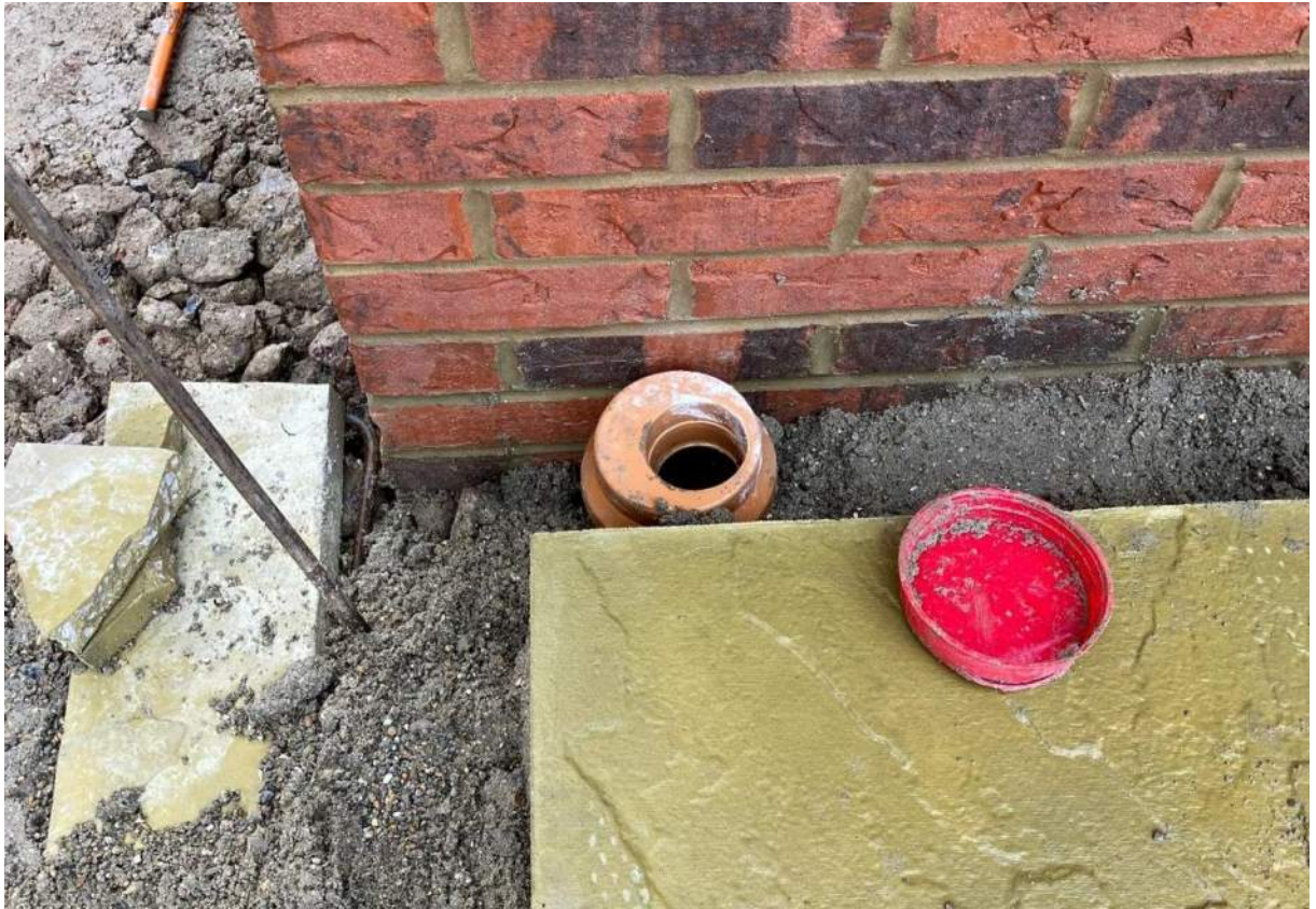
Photo of Rainwater Pipe During Construction
