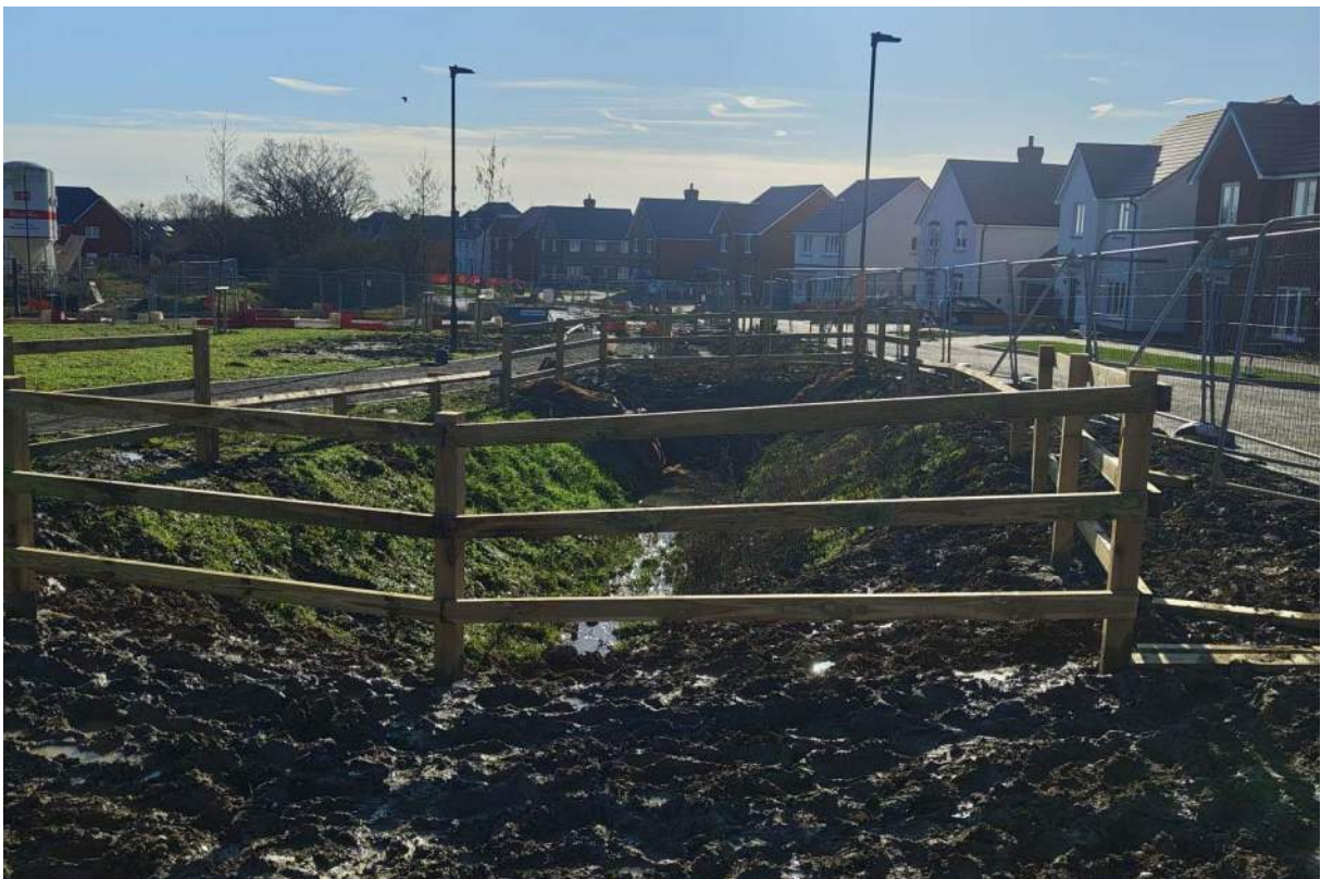
Swale During Construction
