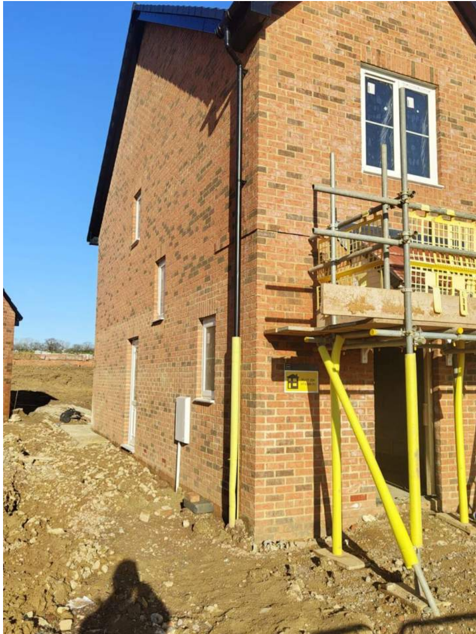
Rainwater Pipe Installed on Site
