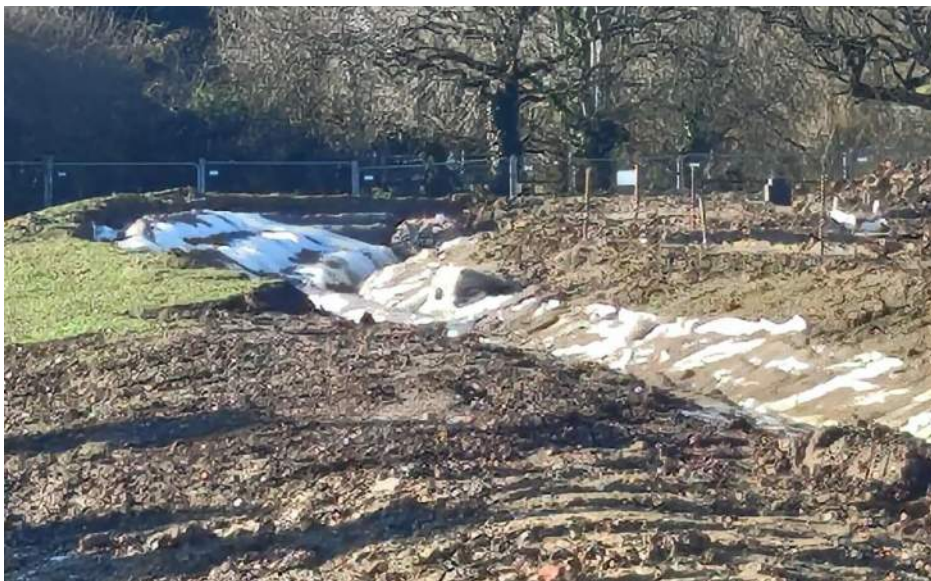
Swale During Construction
