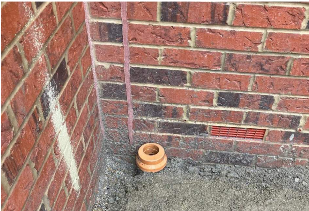
Photo of Rainwater Pipe During Construction
