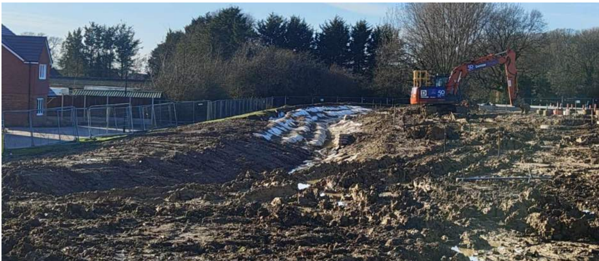
Swale During Construction
