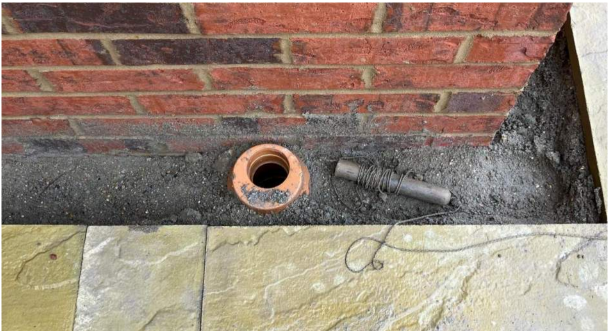
Photo of Rainwater Pipe During Construction
