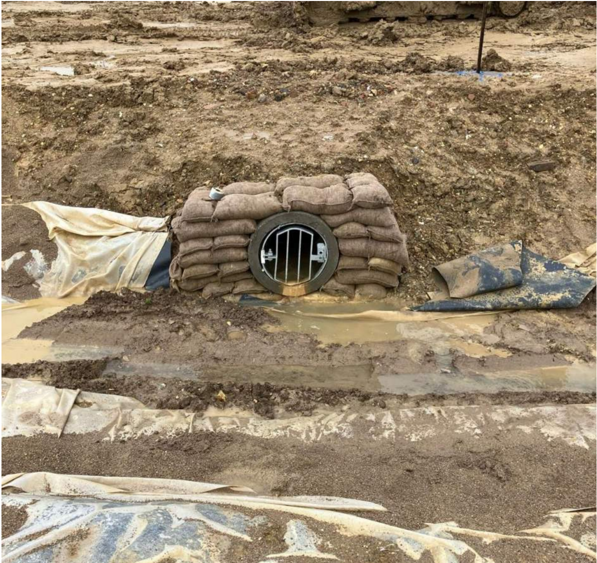
Photo of Concrete Bagwork Headwall During Construction
