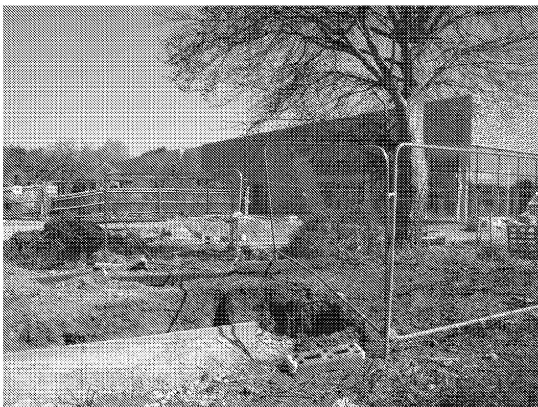
Fig.1 – View NE towards T1
