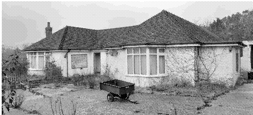
Photo 1 - Block A – Front elevation of bungalow
