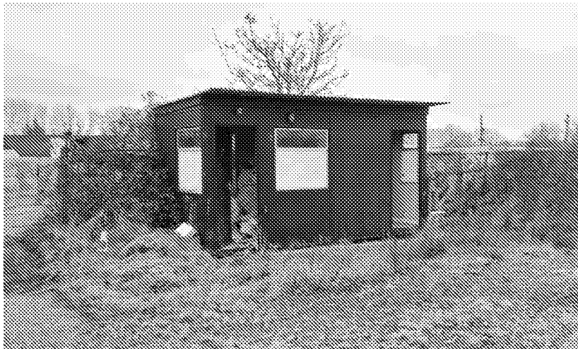
Photo 62 – Block J – View of the hut
