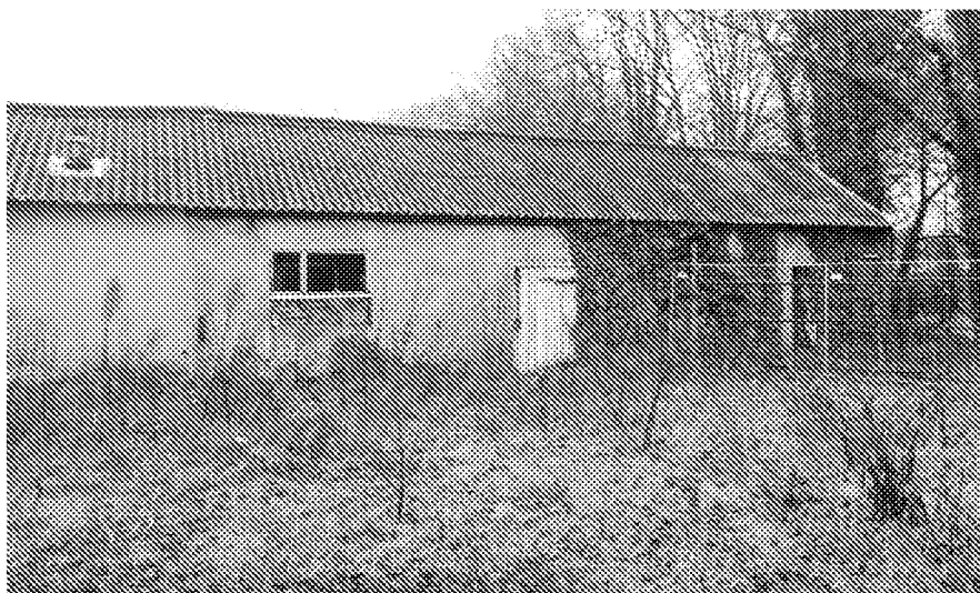
Photo 48 – Block E – View of side elevation
