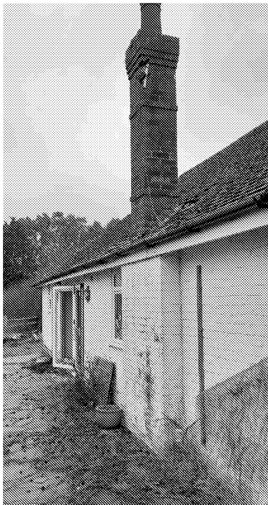
Photo 4 - Block A – Rear elevation showing chimney
