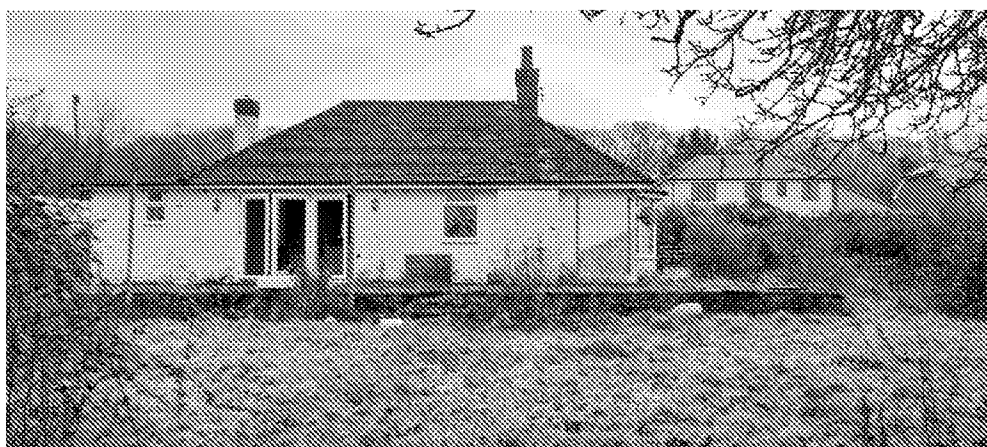
Photo 5 - Block A - Rear elevation showing chimney
