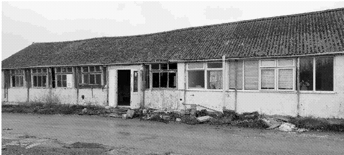
Photo 41 – Block D – Side elevation view
