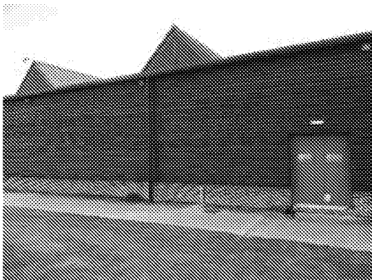
View towards east at rear of Out of Bounds building
