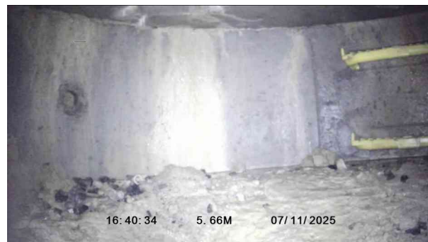
2, 00:00:36, 5.66 m Finish node, manhole, reference: F18
