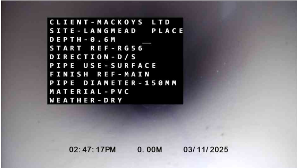
1, 00:00:00, 0.00 m Start node, gully, reference: RG56
