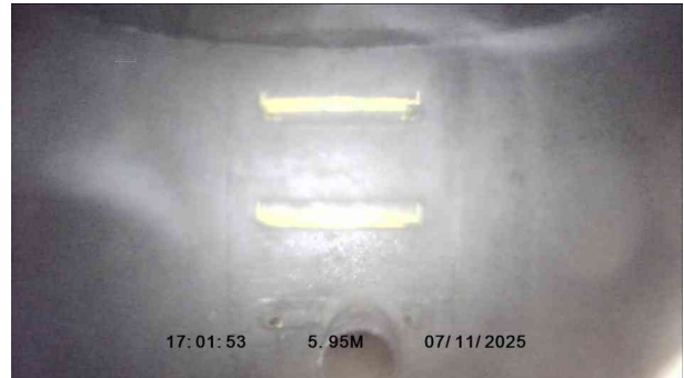
2, 00:00:25, 5.95 m Finish node, manhole, reference: F41
