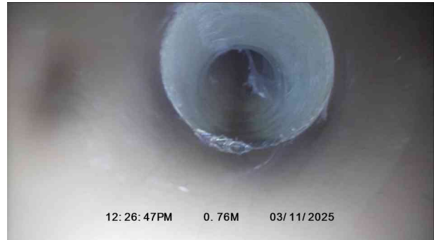
2, 00:00:15, 0.76 m Point repair, localised lining from 12 o'clock to 11 o'clock, start
