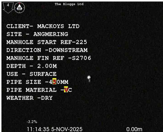
1, 00:00:00, 0.00 m Start node, manhole, reference: 225
