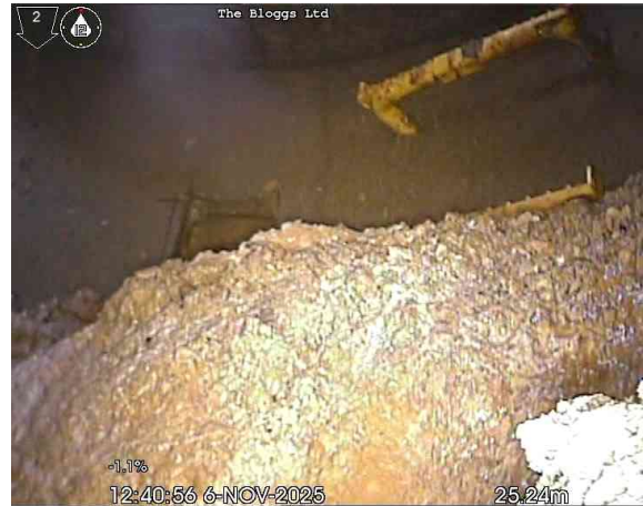
2, 00:02:49, 25.24 m Finish node, manhole, reference: F20
