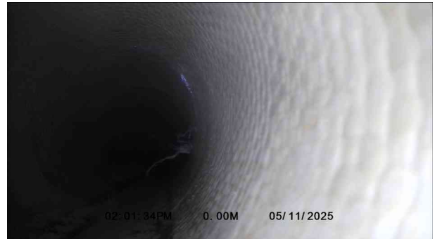
2, 00:00:07, 0.00 m Point repair, localised lining from 12 o'clock to 11 o'clock, start
