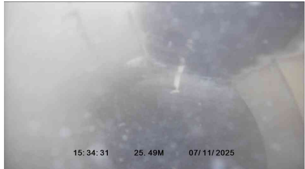
2, 00:01:23, 25.49 m Finish node, manhole, reference: RWP
