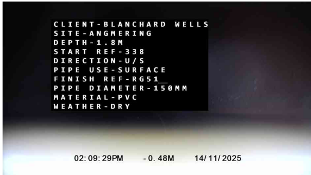
1, 00:00:00, 0.00 m Start node, manhole, reference: 338
