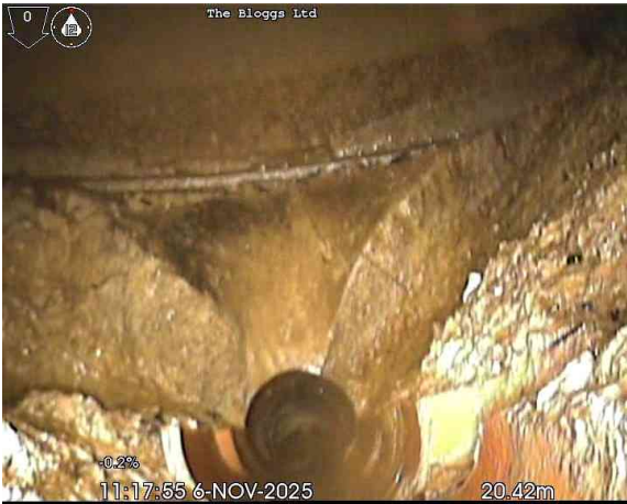
2, 00:02:25, 20.42 m Finish node, manhole, reference: F47
