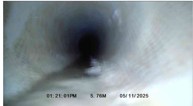
2, 00:00:19, 5.76 m Point repair, localised lining from 12 o'clock to 11 o'clock, start
