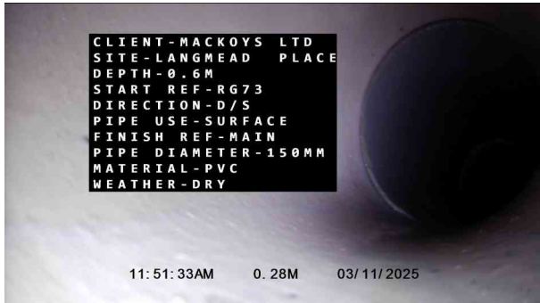
1, 00:00:00, 0.00 m Start node, gully, reference: RG73
