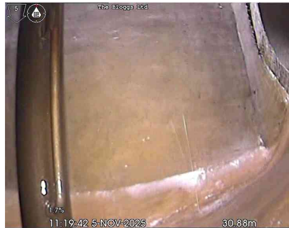
2, 00:03:04, 30.88 m Finish node, manhole, reference: S2706
