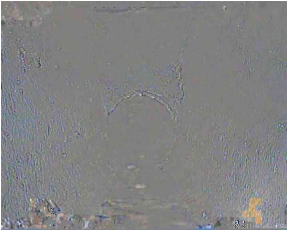
3, 00:02:33, 20.32 m Finish node, manhole, reference: F42
