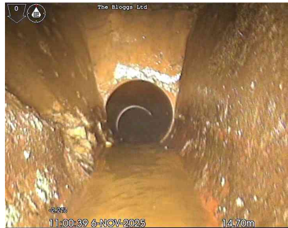
2, 00:01:59, 14.70 m Finish node, manhole, reference: F43
