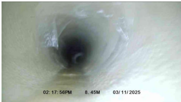
3, 00:00:29, 8.45 m Point repair, localised lining from 12 o'clock to 11 o'clock, start
