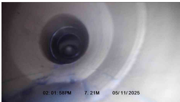
3, 00:00:30, 7.21 m Pipe size changes, new size(s), 100mm high
