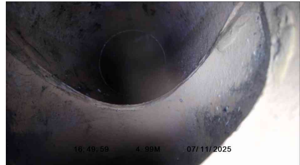
2, 00:00:31, 4.99 m Finish node, manhole, reference: F39
