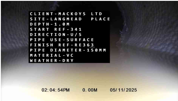
1, 00:00:00, 0.00 m Start node, manhole, reference: 341
