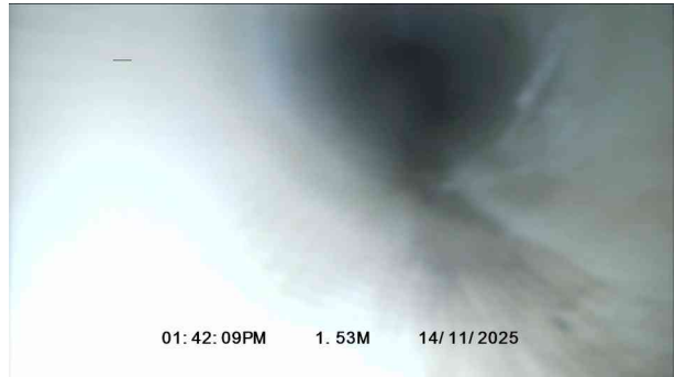
2, 00:00:10, 1.53 m Point repair, localised lining from 12 o'clock to 11 o'clock, start
