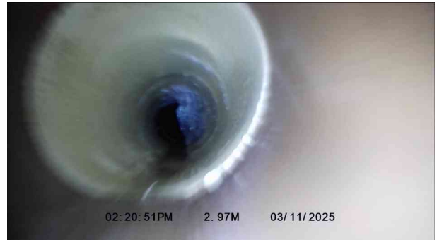
2, 00:00:11, 2.97 m Point repair, localised lining from 12 o'clock to 11 o'clock, start
