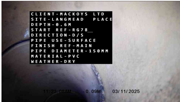
1, 00:00:00, 0.00 m Start node, gully, reference: RG78
