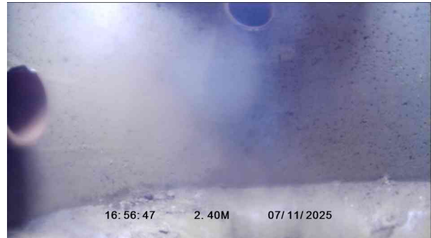
2, 00:00:41, 2.40 m Finish node, manhole, reference: F41
