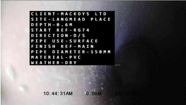
1, 00:00:00, 0.00 m Start node, gully, reference: RG74
