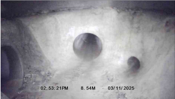
2, 00:00:36, 8.54 m Finish node, manhole, reference: MAIN
