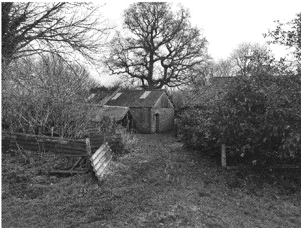
View looking eastwards towards Buildings 1 and 4
