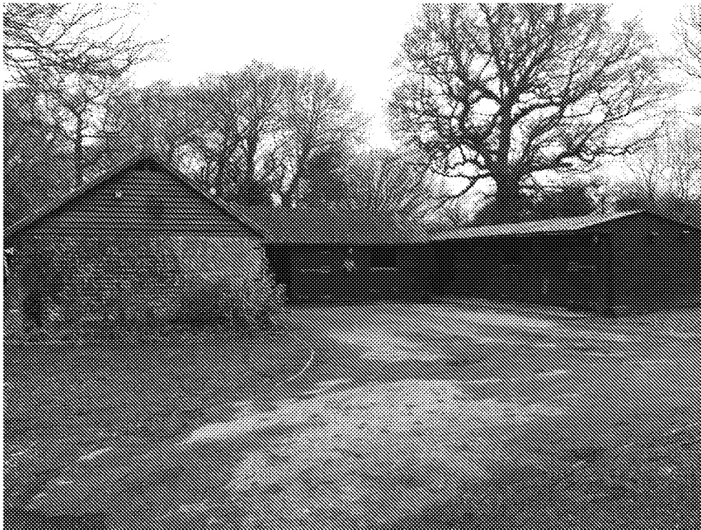
View of Buildings 1, 2 and 3 taken from Decoy Lane looking north-east
