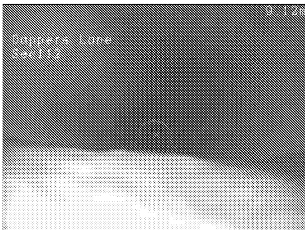
5, 00:00:48, 9.10 m Water level, 30% of the vertical dimension
