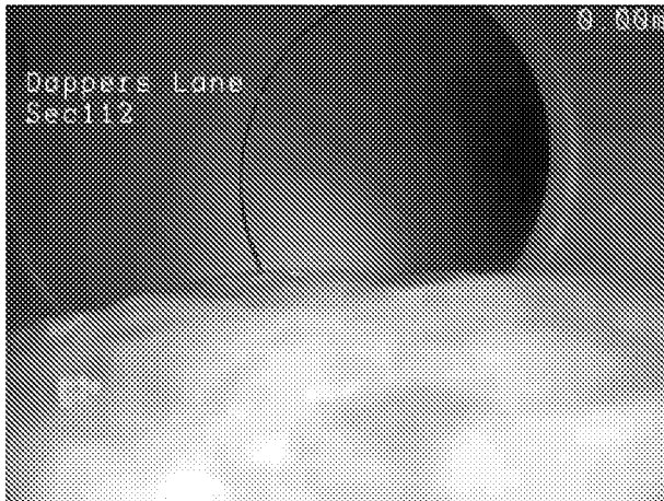
1, 00:00:00, 0.00 m Start node, manhole, reference: S34
