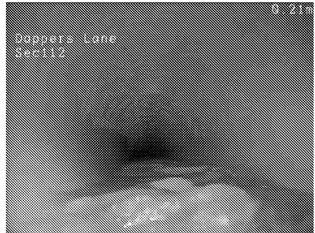
2, 00:00:11, 0.20 m Water level, 20% of the vertical dimension, Live
