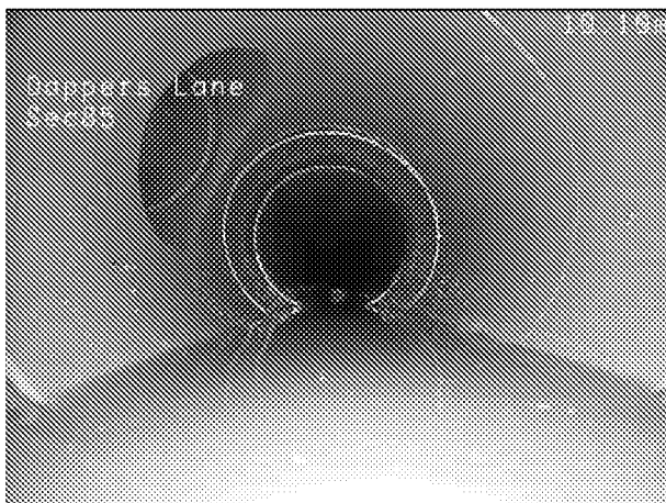
5, 00:00:59, 10.30 m Junction at 10 o'clock, 100mm dia
