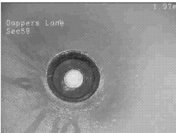
3, 00:00:27, 2.00 m Finish node, manhole, reference: SP41
