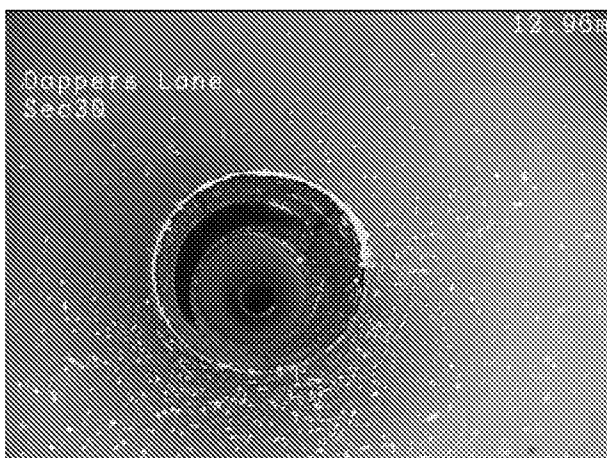
5, 00:00:56, 13.10 m Finish node, manhole, reference: SP22
