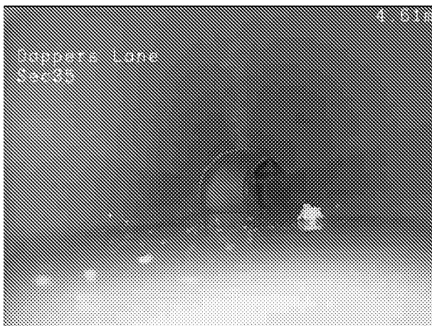
5, 00:00:44, 4.60 m Water level, 40% of the vertical dimension
