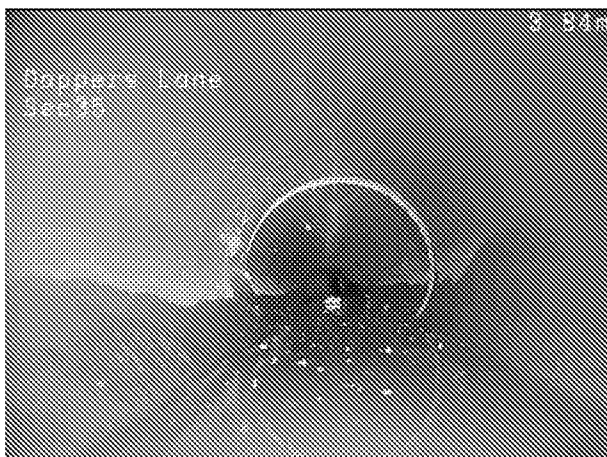
3, 00:00:29, 3.80 m Water level, 15% of the vertical dimension
