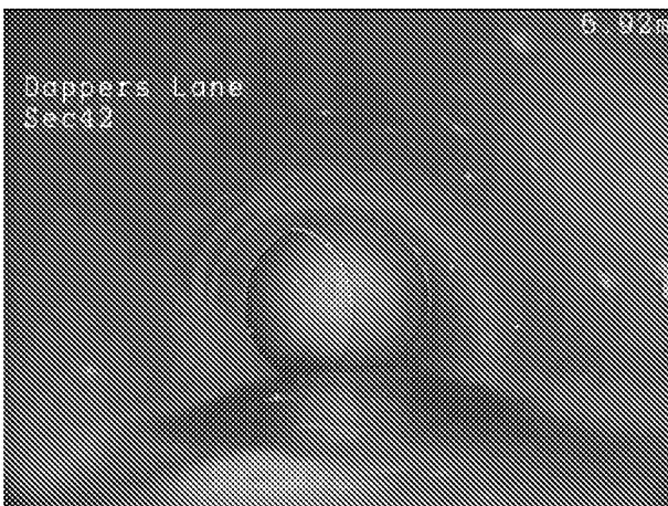
5, 00:00:57, 6.90 m Water level, 10% of the vertical dimension
