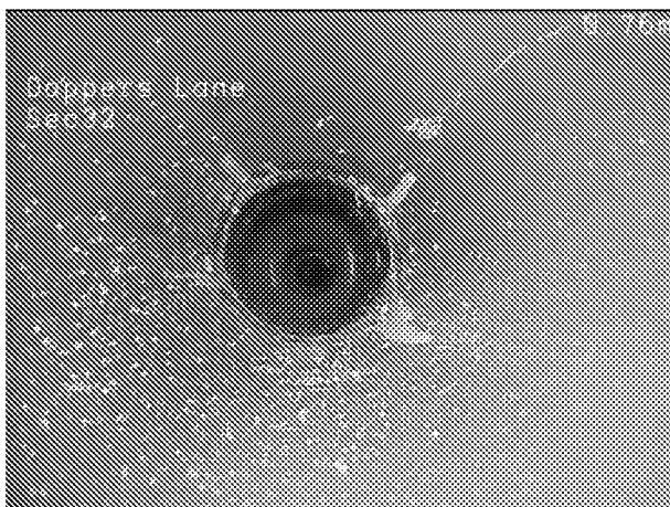
3, 00:00:13, 0.80 m Finish node, manhole, reference: SP23
