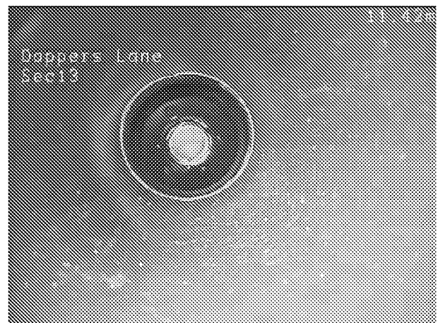
4, 00:00:50, 11.40 m Finish node, manhole, reference: SP10
