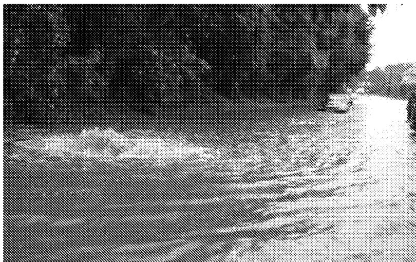
Plate 7.2: Evidence of the surface water sewer surcharging in Water Lane (date photo was taken is not known).
