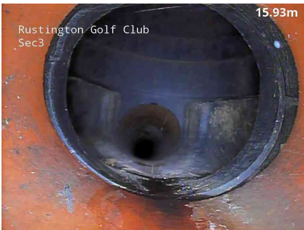
5, 00:00:09, 16.20 m Finish node, manhole, reference: SW2
