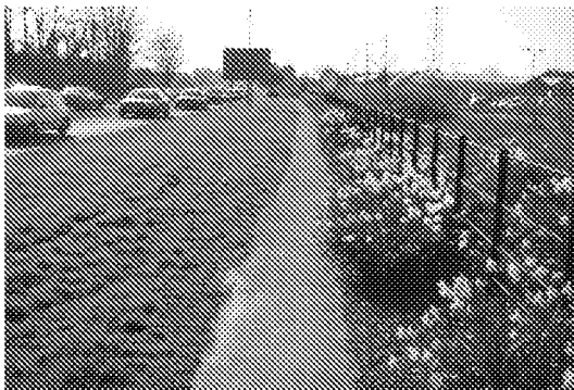
Figure 3.5: Footway infrastructure on the A259
