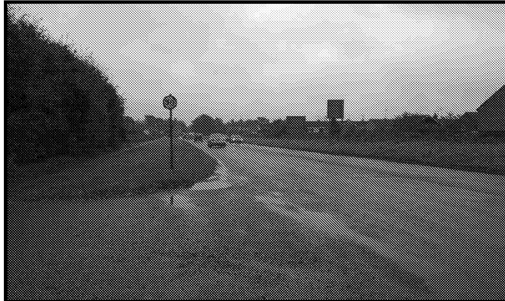
Figure 10: Photo of existing southern access onto A259
