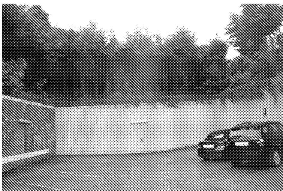
Plate 4. Truncation associated with building of the garage complex looking south-east
