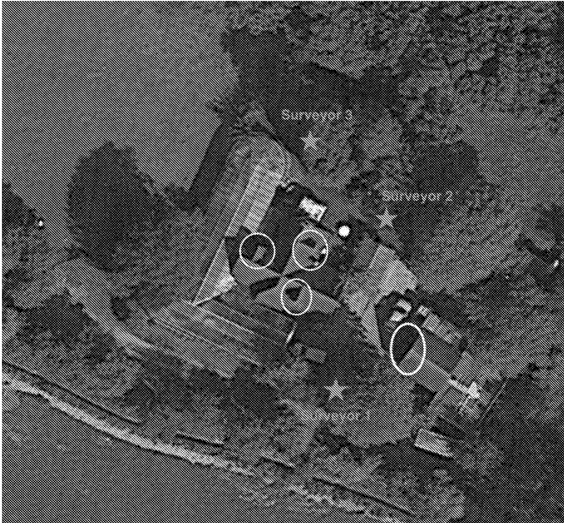
Figure 2: Surveyor positions around the house to cover all areas of interest (Yellow circles indicate areas of lifted weatherboarding)
